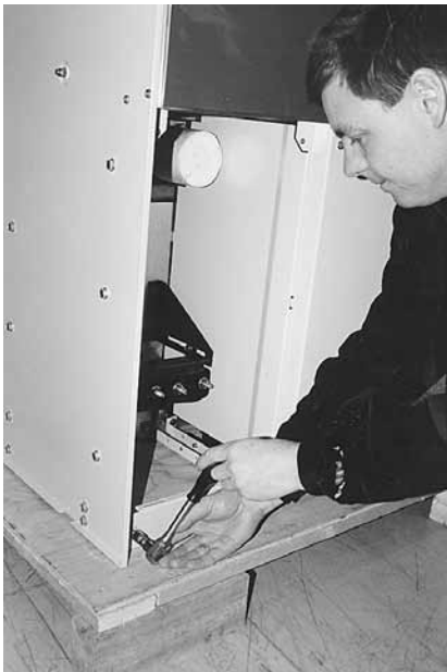
2. Removal of front section.
