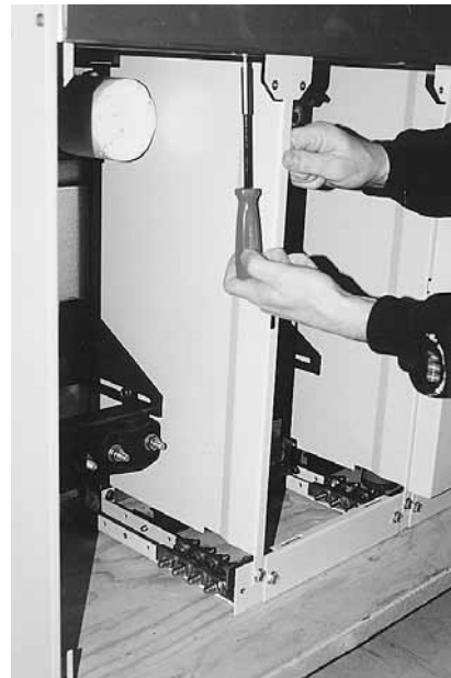
4. The panel can be removed by unscrewing A and B.
