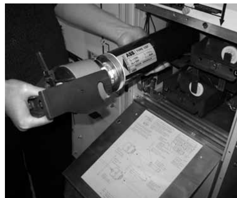
6. Pull out the fuse handle. The fuses are firmly fixed in the fuse cover.
